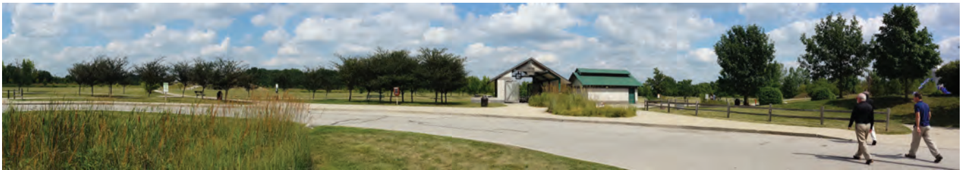
Photo 2-5. View of Shelter and Toilet Buildings
