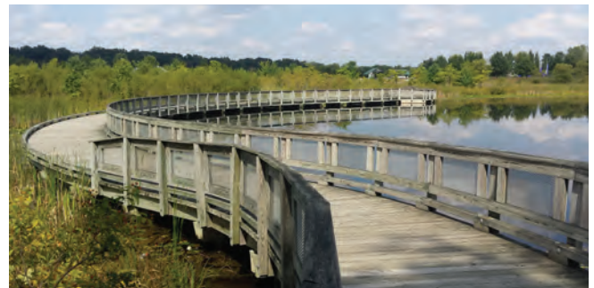
Photo 2-11. Existing Wetland Boardwalk
