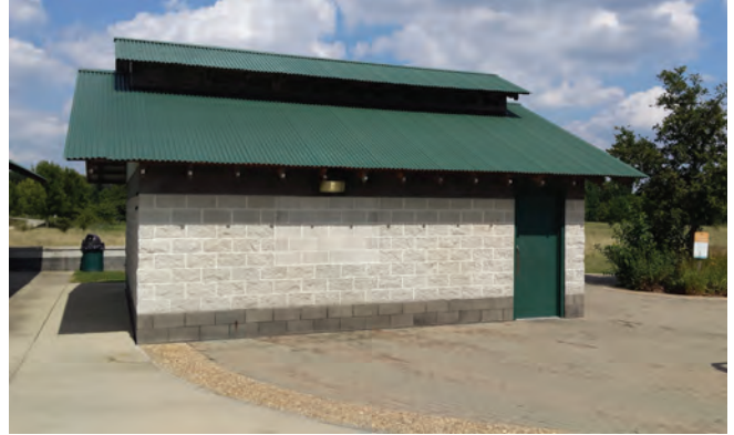
Photo 2-13. Existing Restroom Building
