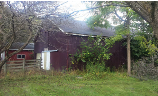
Photo 2-16. Existing Barn, The Groves
