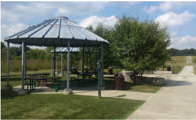
Photo 2-14. Existing Silo Shelters
