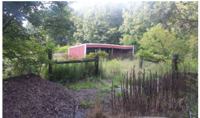
Photo 2-17. Existing Structure, The Groves
