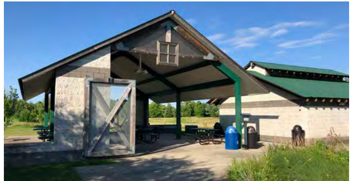
Main shelter and restrooms
