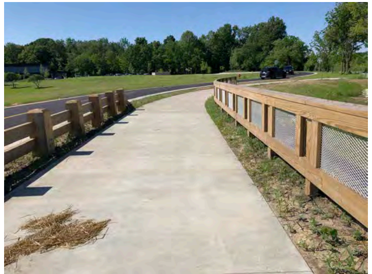
Vehicular and pedestrian guardrails at the Groves
