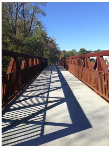
Bridge Along Trail
