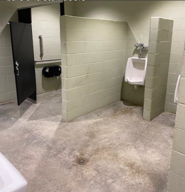
Toilet seat and bowl, toilet and urinal sensors, toilet paper dispenser, grab bars and stall doors
