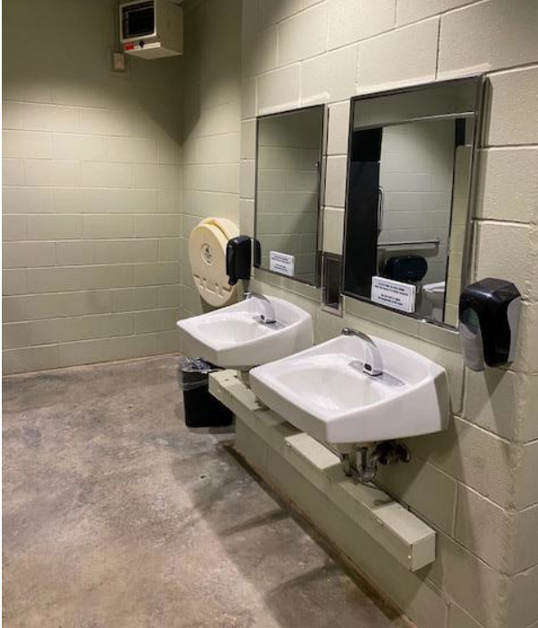
Hand soap units, faucets, sinks, and changing table
