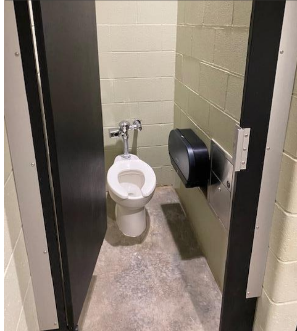
Toilet seat and bowl, toilet sensor, toilet paper dispenser, sanitary disposal and stall doors
