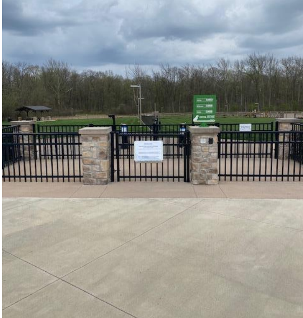
Gates entrances on either side of bullpen and key fob scanners
