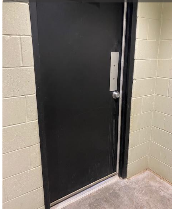
Door handle plate and inside of door
