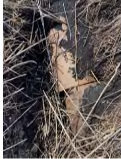
Figure 5: Drainage tile blowout
