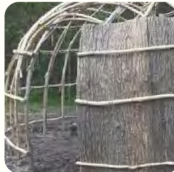
BUILDING METHODS: BENT SAPLINGS/POLES & THIN BARK COVERING Source: http://www.woodlandindianedu.com/wigwamlonghouse/longhouse.html
