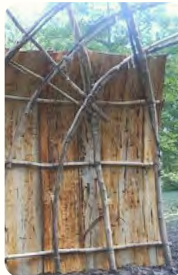
BUILDING METHODS: BENT SAPLINGS/POLES & THIN BARK COVERING Source: http://www.woodlandindianedu.com/wigwamlonghouse/longhouse.html
